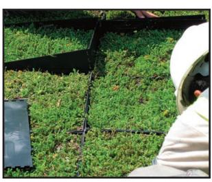
Removing sides allows plant material to grow together.
